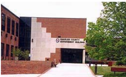
Commissioners Gallery Charles County Government Building
